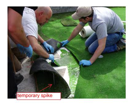
Glue being added to seaming tape. Note temporary spikes being used to hold grass in place while lining up seams.
